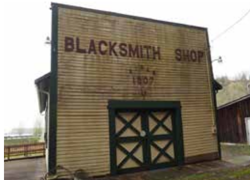
Blacksmith Shop, Stella, WA
